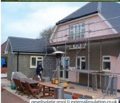
gevelisolatie resol © externalinsulation.co.uk
